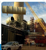
Big diameter ducts, chimneys or tanks: on-site welded
